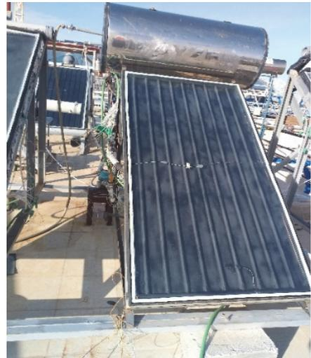
*Solar water flat plate solar collector*
