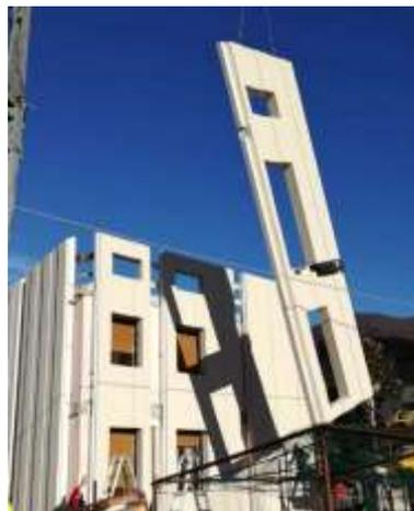
Figure 7: Installation of a fully OSC solution (Woodbeton, 2023)
