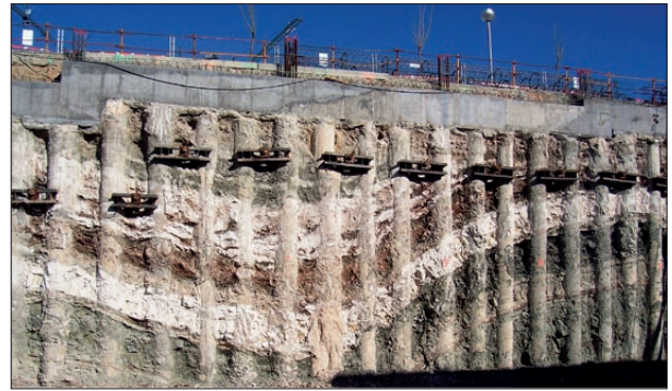
Fig. 6: Areas with folding and softened clay.
