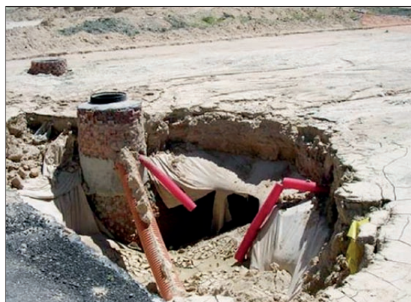
Fig. 12: Damages to a collector caused by broken pipes.
