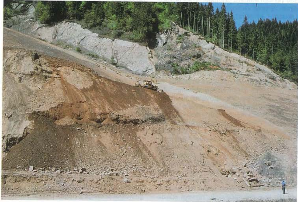
Dela na odkopavanju in izravnavanju površine plazne gmote (Foto A. Horvat) Excavation and levelling work on the area of landslide material (by A. Horvat)
