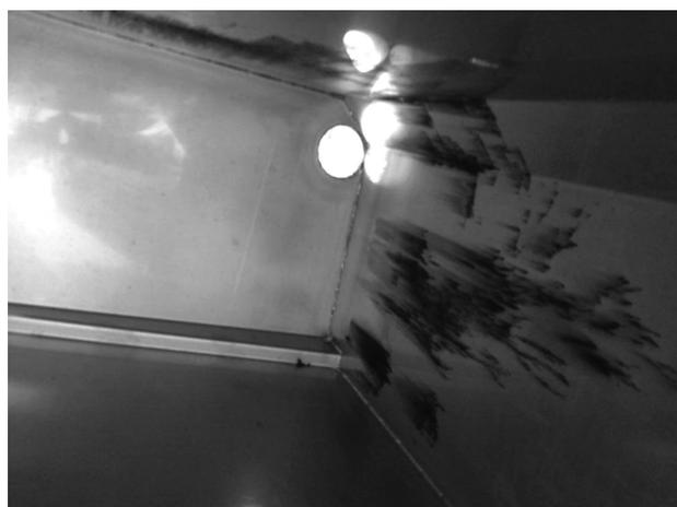
**Figure 2:** Local corrosion damage inside the tank
