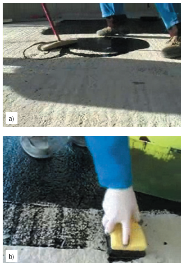
Fig. 2. Testing of the working principle for a) circular spreading of the hydro insulation material with a brush and b) pressing it with a sponge
