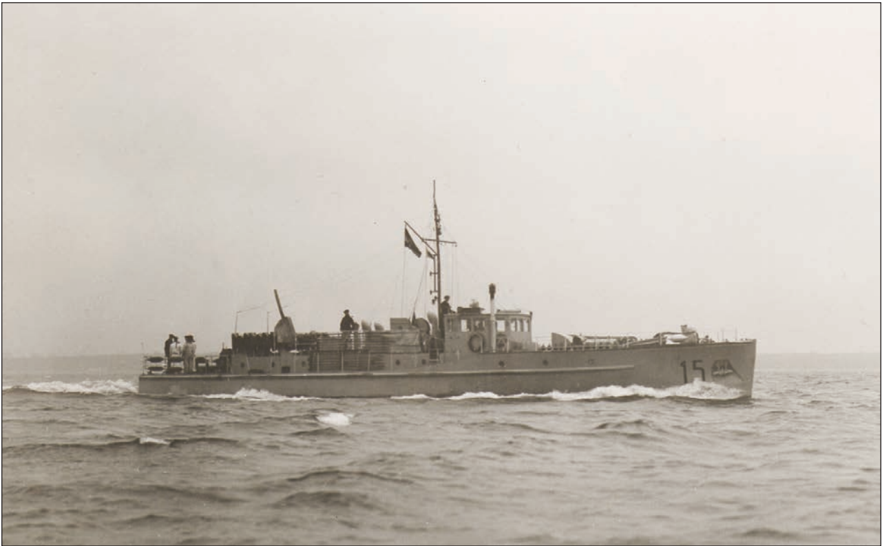
Figure 1: German light minesweeper (Minen-Räumboot) R 15 on the North Sea on 5 November 1934. Length (LOA) 27.75 m; beam 4.38 m; depth 2.15 m; draught 1.36 m; displacement 52.5 t (Source: Sammlung Dressler, Württembergische Landesbibliothek, Stuttgart; Bildarchiv: 18-0701-a).
