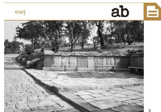
Slika 3 Oblikovanje poti in obnova cerkve svetega Dimitrija Loumbardiarisa na griču Filopap, Atene, Dimitris Pikionis, 1951-1957, foto Akos Moravanszky Figure 3 - Walkway arrangement and Church of St Dimitrios Loumbardiaris renovation, Philopappos Hill, Athens, by Dimitris Pikionis 1951-1957, photo by Akos Moravanszky.
