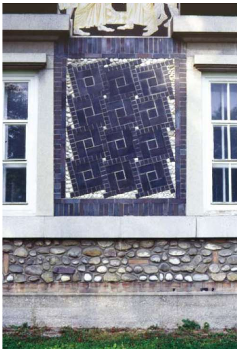
Primer: V kamnu in opeki izveden tekstilni vzorec na Žalah Example: Textile pattern executed in brick and stone at the Žale cemetery in Ljubljana.
