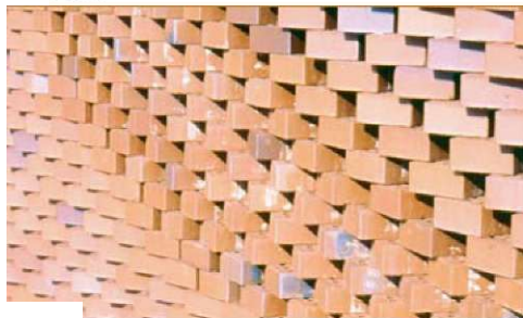
Slika 9: Opečnati zid, ki ga je naredil robot, Studio Fabio Gramazio, Matthias Kohler, ETH Zürich Figure 9: Robot-laid brick wall, Studio Fabio Gramazio, Matthias Kohler, ETH Zürich.
