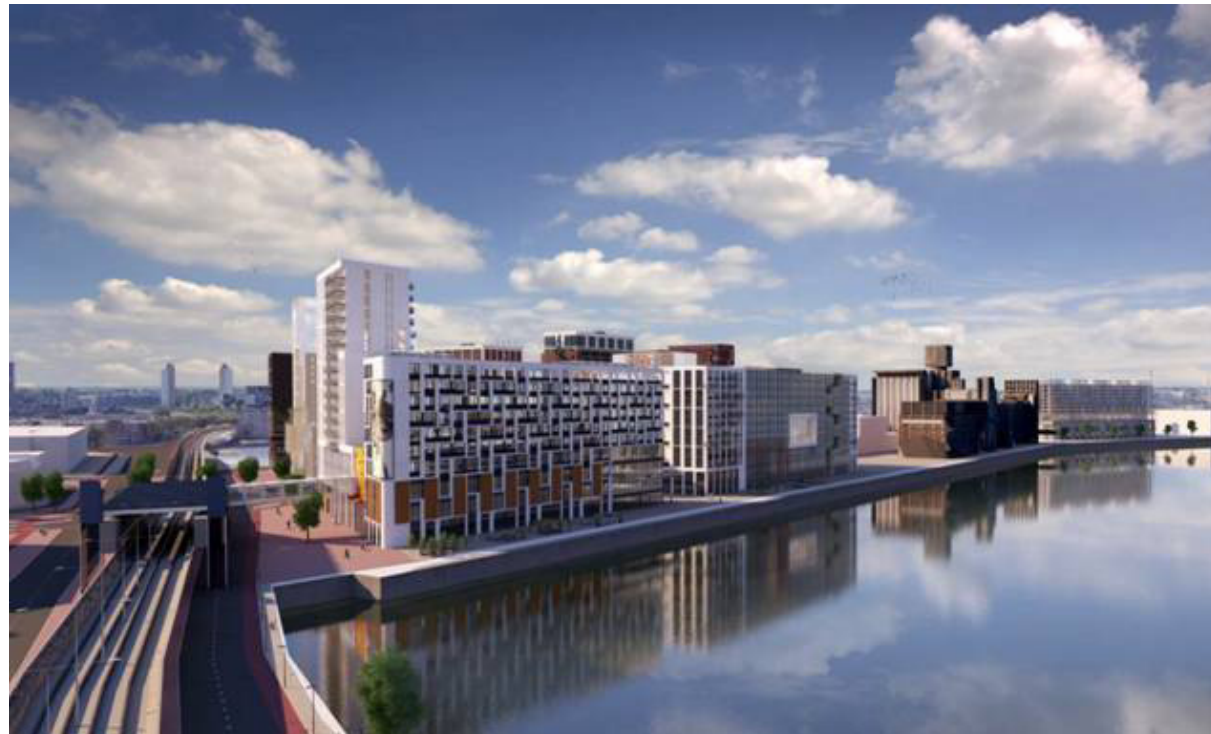
Fig. 16. Joke Vos Architecten, 'The View of Rotterdam' (design update 2017). Photograph courtesy Joke Vos Architecten.
