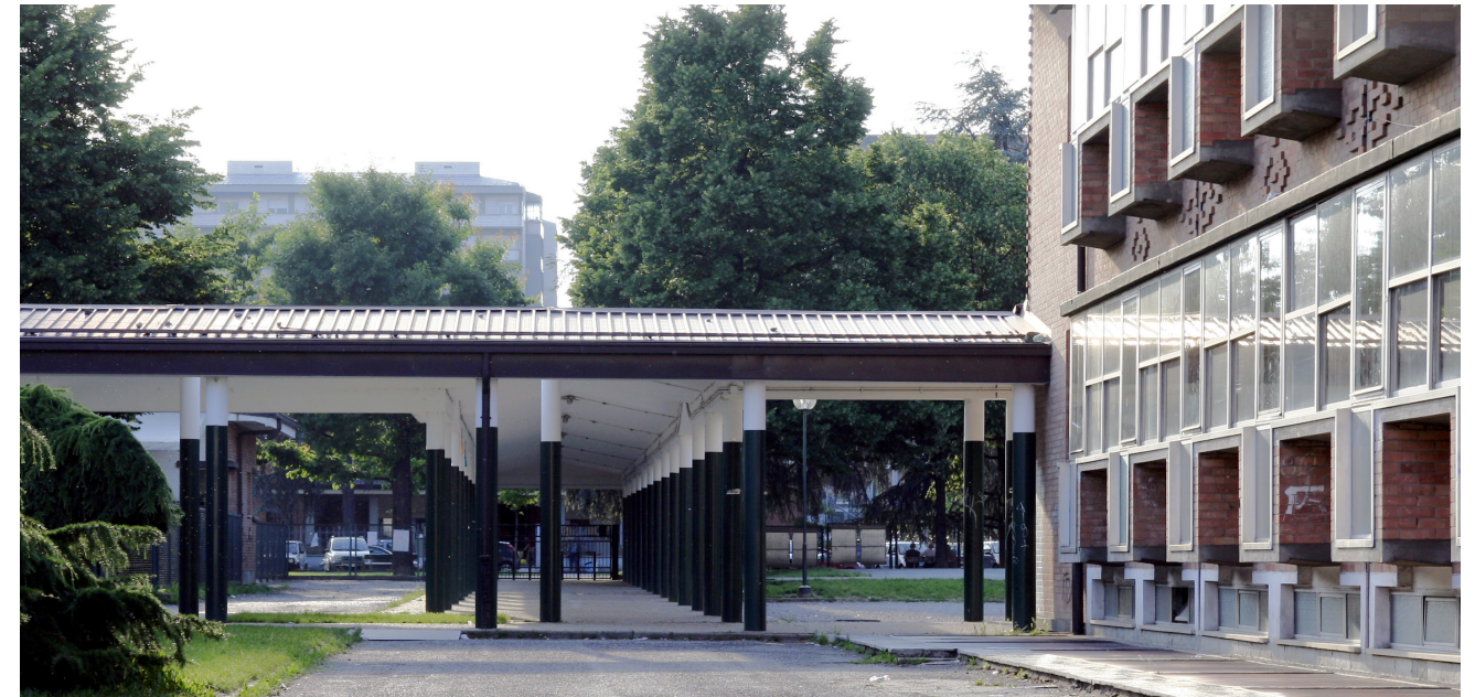
Fig. 9. Ada Bursi, School in via Duino, Turin 1969. Photo by Caterina Franchini.
