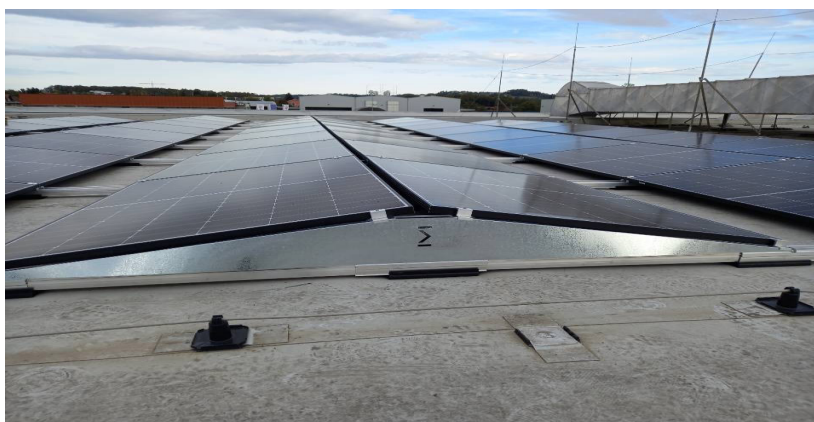
Figure 7: Practical placement of East-West oriented solar modules (own photo)
