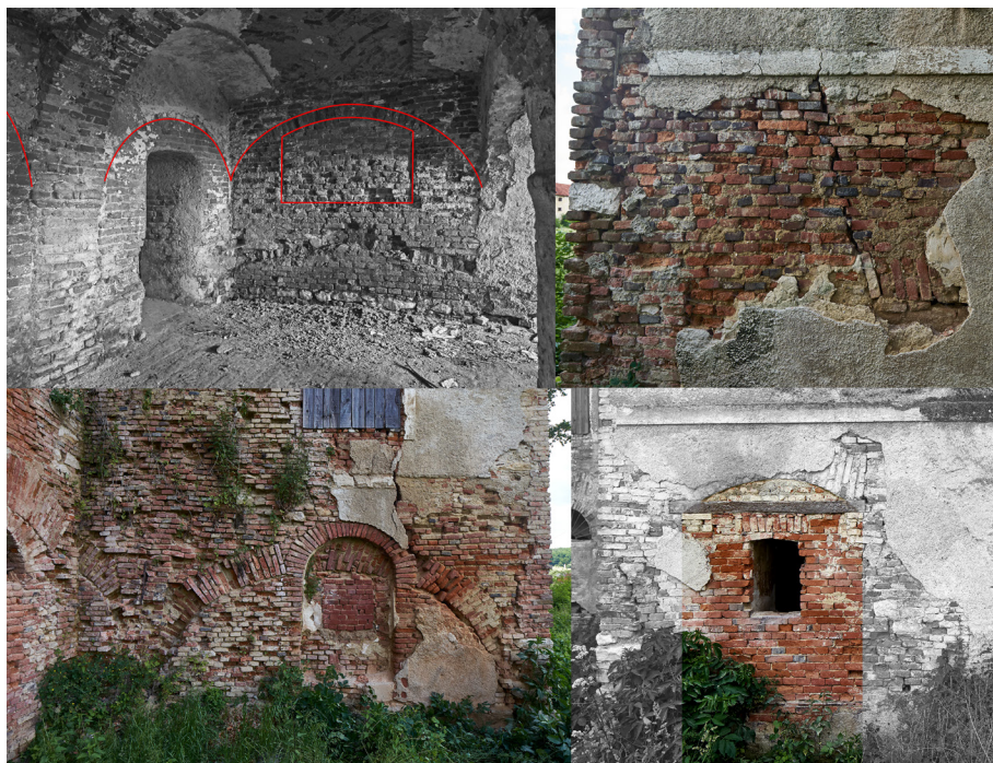
Fig. 5: Poznanovec, Sermage Mansion, southwestern portion of the rectangular ground-floor room believed to be a part of the original core (above left); built-in window and traces of an earlier plaster layer in the ground-floor of the northern part of the western façade (above right); ground-floor of eastern façade of western projection (below left); part of southern façade of western projection (below right), photo: J. Rasol, 2016.; print: R. Mavar, 2016.
