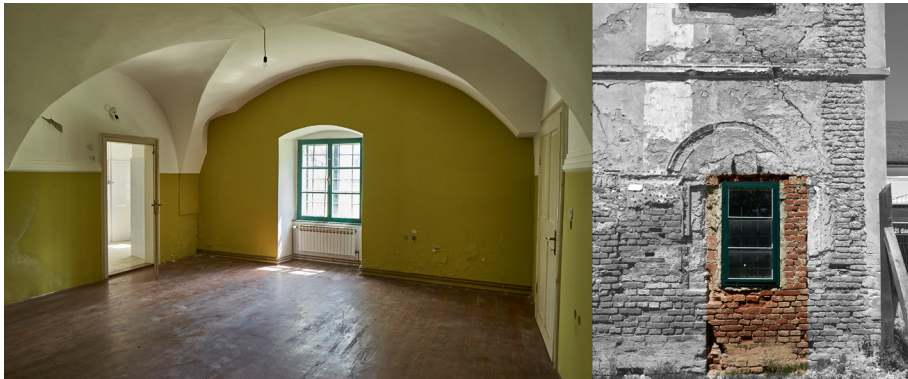
Fig. 4: Veliki Bukovec, Drašković Mansion, cut in vault next to the eastern wall of the rectangular room of the presumed original core (left); built-in entrance to the presumed original core (right), photo: J. Rasol, 2016.; print R. Mavar.
