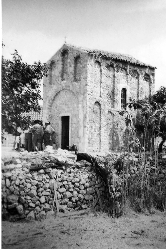
Fig. 4: Ston, Church of St Michael, before restoration, 1921 (Konzervatorski zavod, Odjel u Splitu, Ministarstvo RH).
