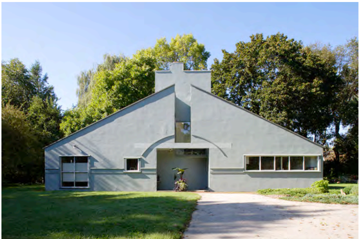
Vanna Venturi House, Philadelphia, Pennsylvania, 1964 Photo by Matt Wargo
