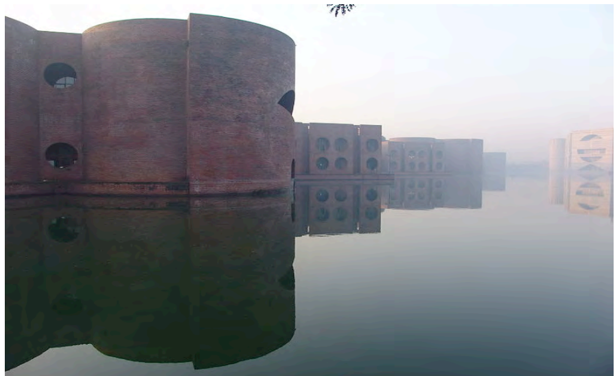
zgoraj- Salk Institute, La Jolla, California 1959, v sredini levo Richard Medical Centre 1961, desno Escheric House, 1961, spodaj National Essembly Dacca, 1974
