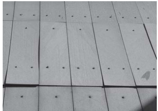
Figure 5. Bowing on the south facade of neighbouring building
