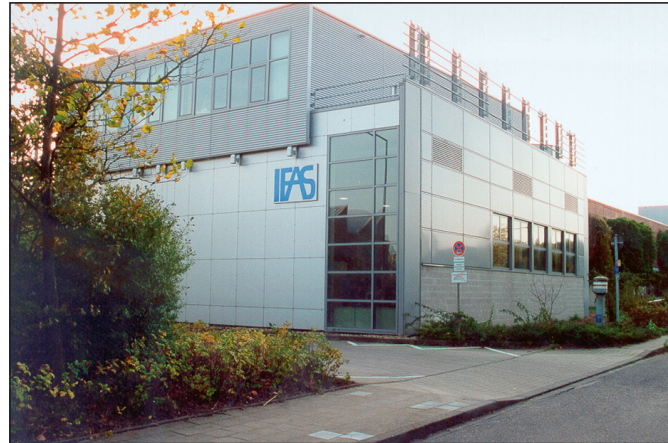
IFAS – Main building
