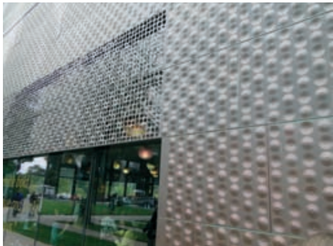
Slika 9: Perforirana in reliefno oblikovana bakrena pločevina na fasadi (Muzej mladih, San Francisco, Herzog & de Meuron 2005) [Foto: Zbašnik-Senegačnik]. Figure 9: Perforated and relief copper sheet metal on a façade (The de Young Museum, San Francisco, Herzog & de Meuron, 2005) [Photo: Zbašnik-Senegačnik].
