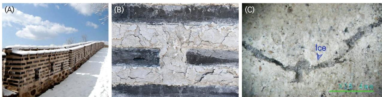
**Figure 1:** Damage to Namhansanseong Mock Yeojang (Parapet) due to freeze-thaw: a) Namhansanseong Yeojang (Parapet) in winter (Gyeonggi Cultural Foundation website), b) detailed photograph of the surface of Namhansanseong Mock Yeojaing (Parapet) damaged by freeze-thaw, c) ice inside the surface crack of Namhansanseong Mock Yeojang (Parapet)
