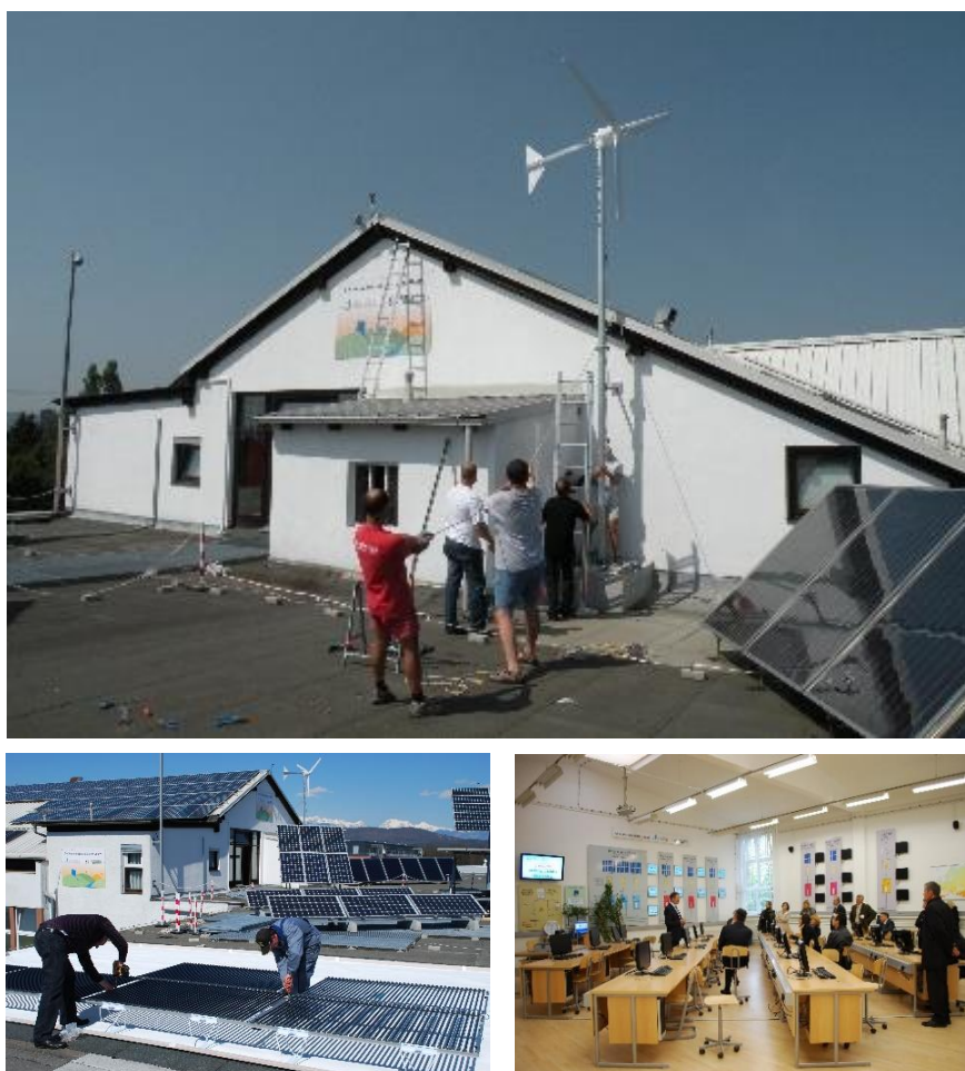
Spletna kamera, vetrni in toplotni generator, cevni PV-generator in nadgrajeni monitoring.
