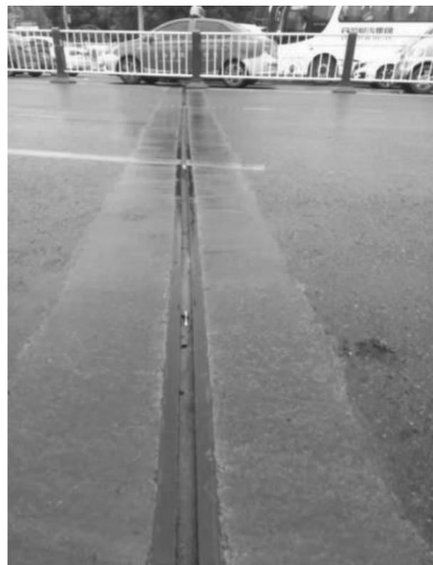
**Figure 9:** BECI of the Jihe Bridge using the steel-PVA hybrid fiber concrete
