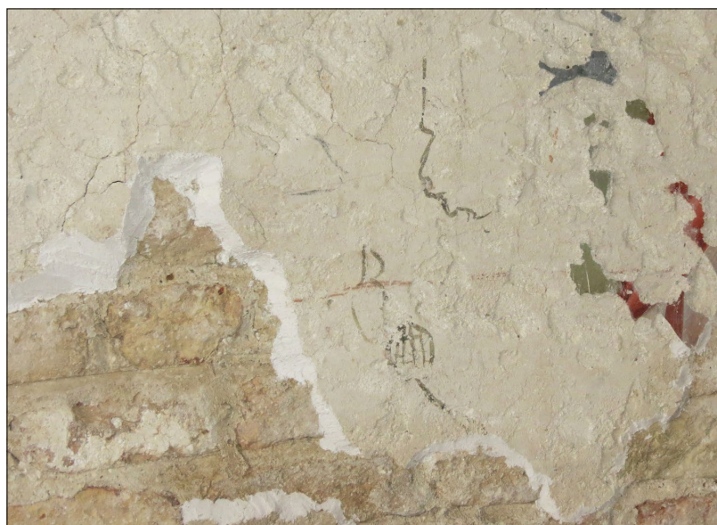
9. A red line of sinopia , drawn on arriccio in a red ellipse. St Francis of Assisi church in Koper (Photo: Anabelle Križnar).
