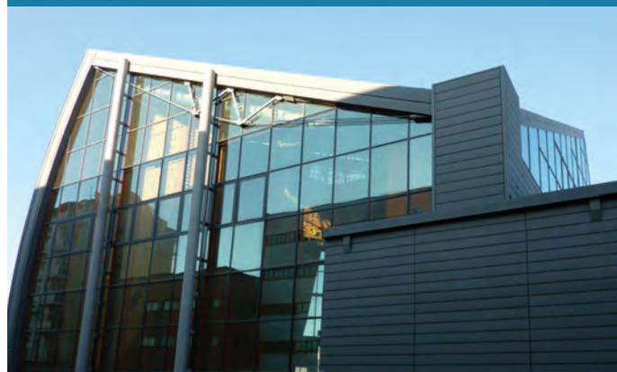
tensioned beams in laminated wood that is hinged to a single reinforced concrete pillar and braced by the metal cylinder of the lift shaft. The exterior side facing the street is entirely glazed, thus making the climbers visible day and night. The roofing and part of the façades are coated with grey zinc-titanium which evokes the colours of the mountains, while the interior space
