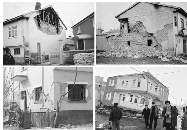
Figure 1: Some damaged masonry buildings 14 (Sultandagi-Cay Earthquake, 2002)
