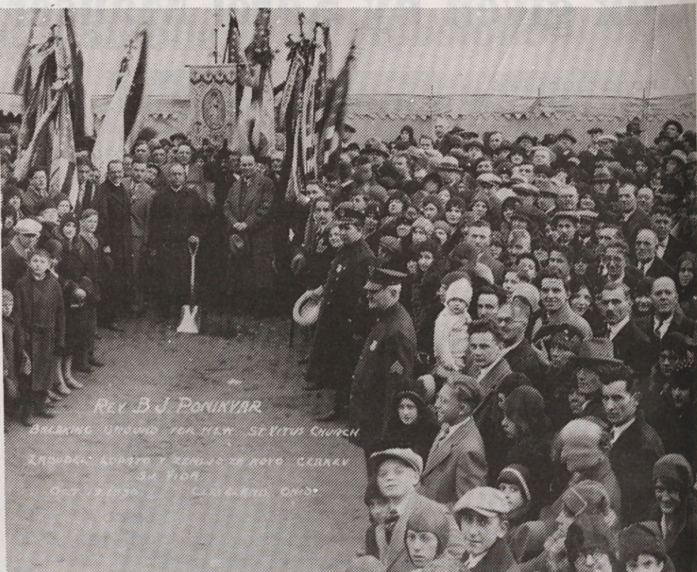
Rev. B. J. Ponikvar breaking ground for new St. Vitus Church on October 19, 1930, Cleveland, Ohio
