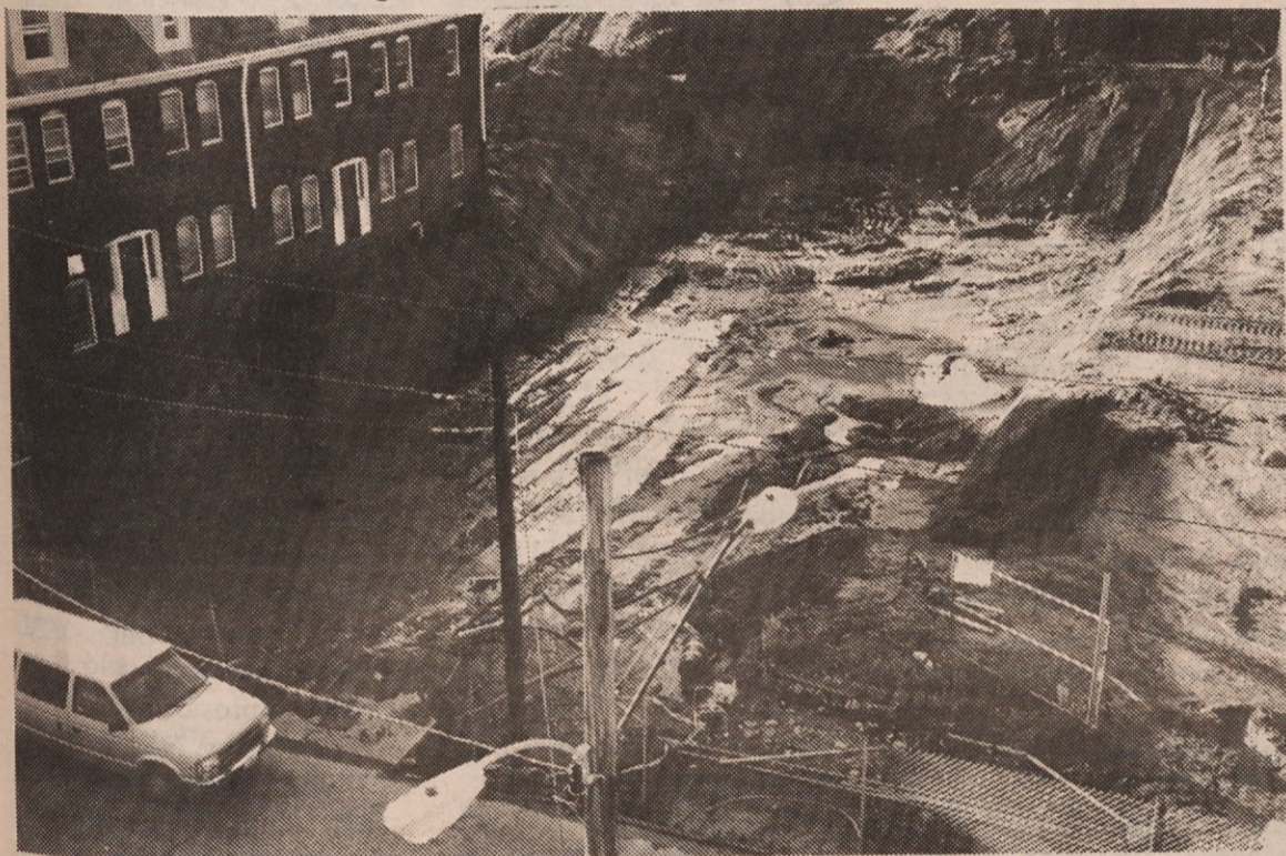
St. Vitus Village excavation site facing Glass Avenue. Land is being removed to make way for the basement portion. The brick building on the left is scheduled for demolition in early October.
