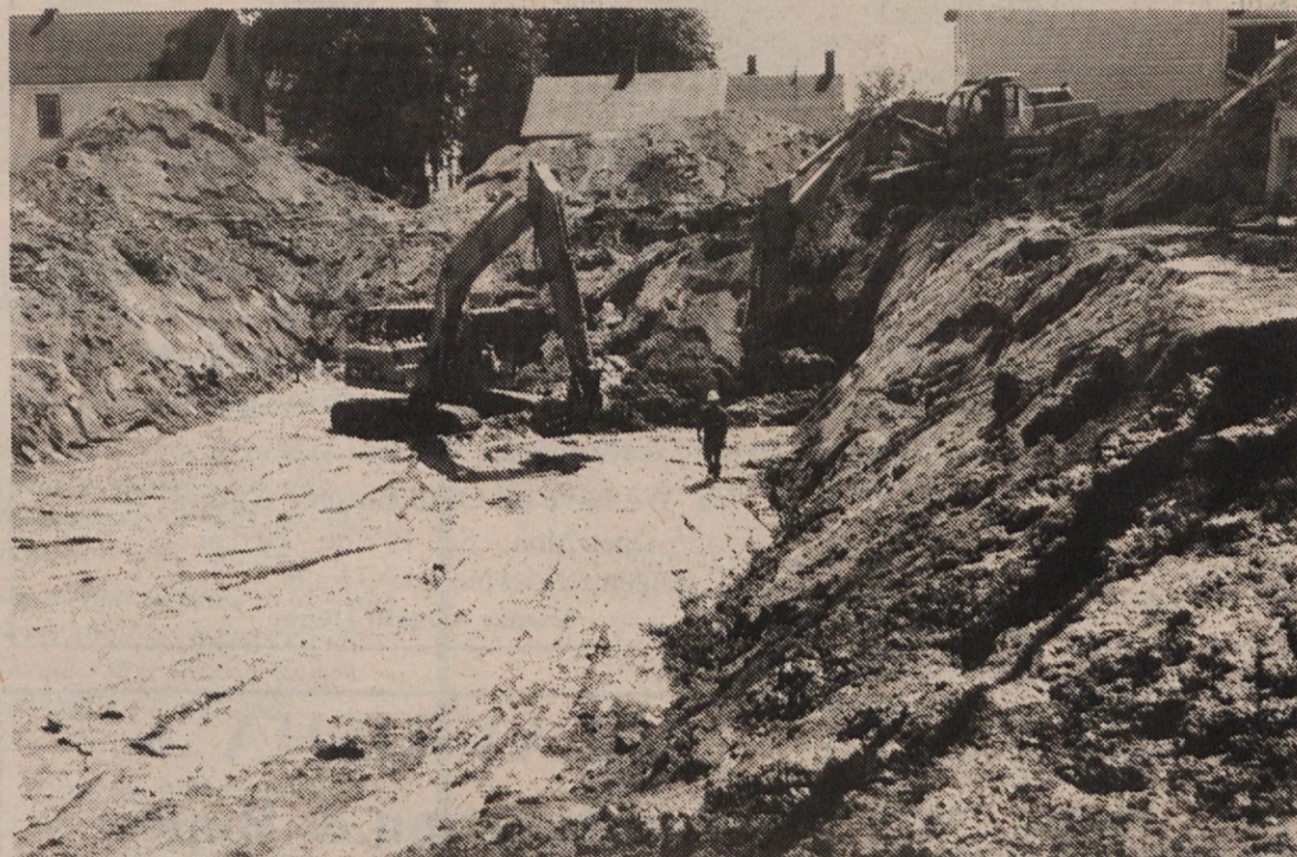
Facing East 61 st Street. Area here is the former St. Vitus Convent. This will be a direct drive-in garage parking for 11 spaces. Remaining 22 car spaces will be outdoors by the court-yard.
