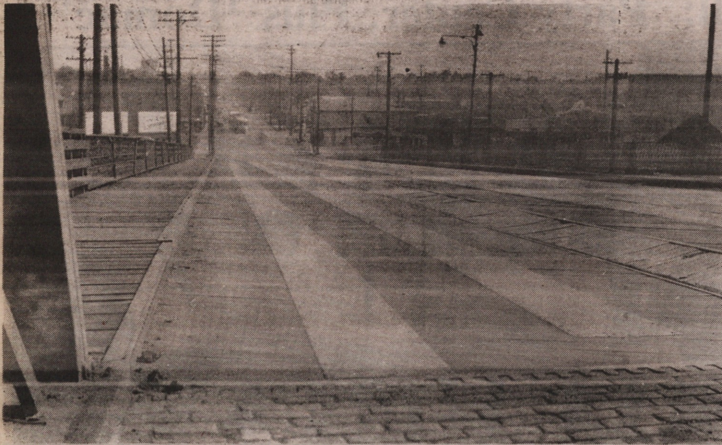
Collinwood Bridge in 1930s. Note wooden planks and rails for streetcars and the road which is paved with bricks. A streetcar can be seen at the bottom of the bridge, upper left. The bridge went over the Collinwood New York Central Railroad yard where a roundhouse and switching yard
