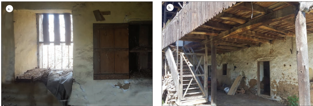
Figure 12: A traditional house in Janchishte, Tetovo: a) the wide parapet of a window; b) the floor with wooden planks and beams above the hajat (Photo: Aurora Saidi).
