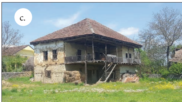
Figure 8: An example of the çardak and the qyshk in a traditional house in Tetovo: a) A traditional house in Poroj, Tetovo (personal archives of the respondents); b) The qyshk in the çardak (personal archives of the respondents); c) A traditional house in Janchishte, Tetovo (Photo: Aurora Saidi).
