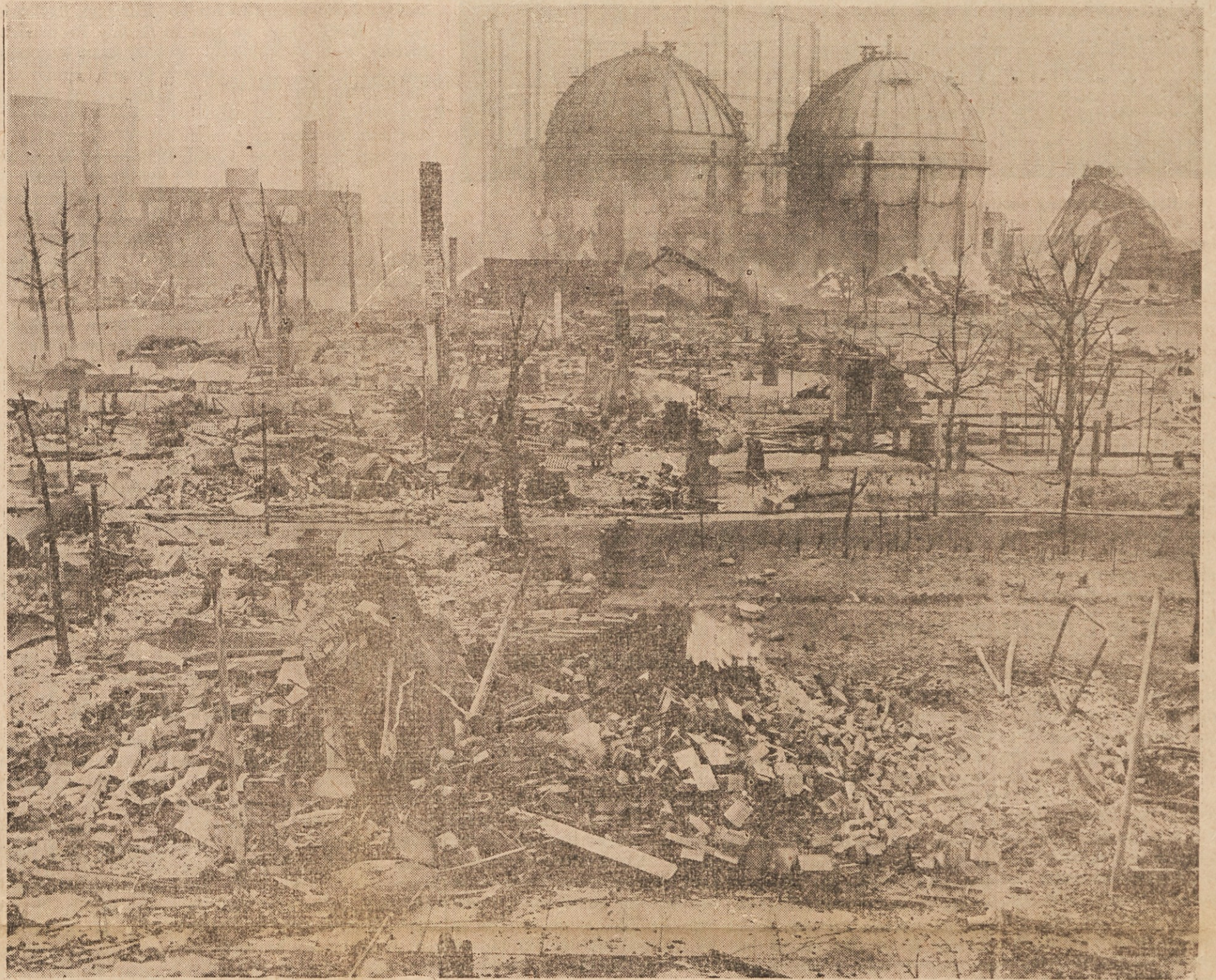
Scene of total devastation of E. 61st Street north of St. Clair. Collapsed gas tank can be seen in right hand corner of picture.
