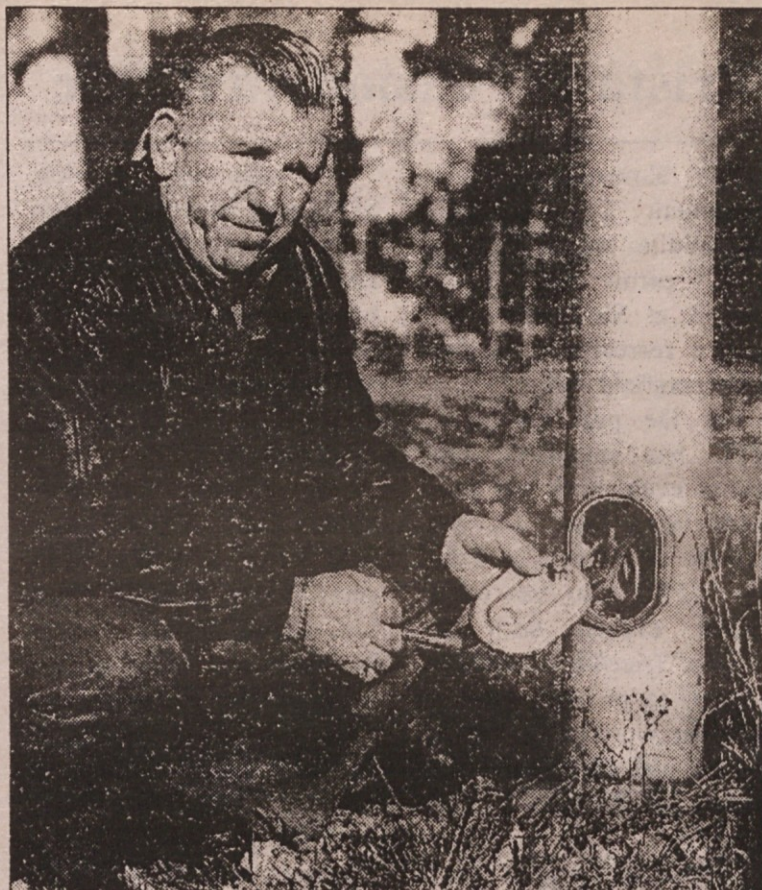
ROBERT A. DAVIS SUN-TIMES Jure Pozek displays the device that he says makes it virtually impossible for criminals to cut the wiring in the base of a street light.
