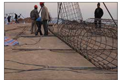
(c) Make of reinforcement cage
