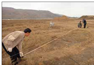
(a) Preparation for construction
