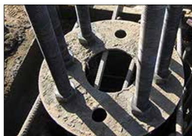
(e) Installation of locking nut
