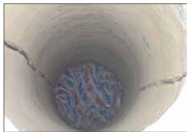
(b) Excavation of borehole
