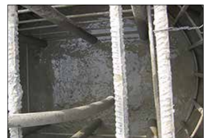
(f) Pouring of concrete
