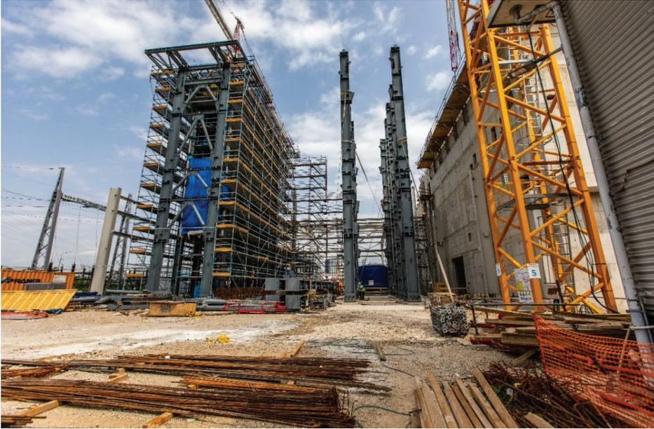
**Figure 5:** The HRSG casing steel structure
