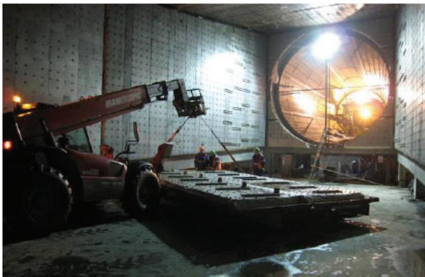
*Figure 8: The HRSG inlet duct erection*
