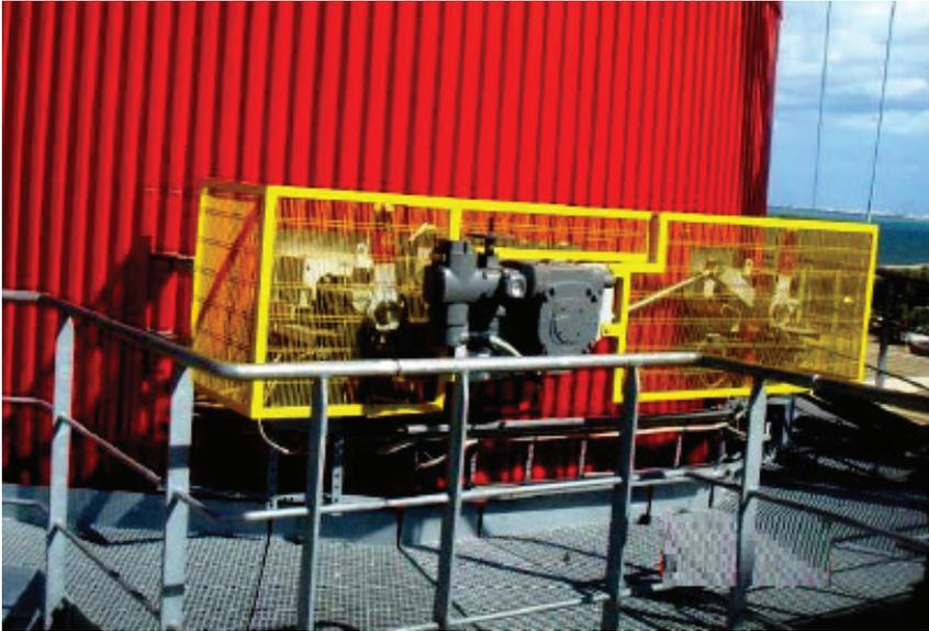
*Figure 10: The HRSG water dumper drive*
