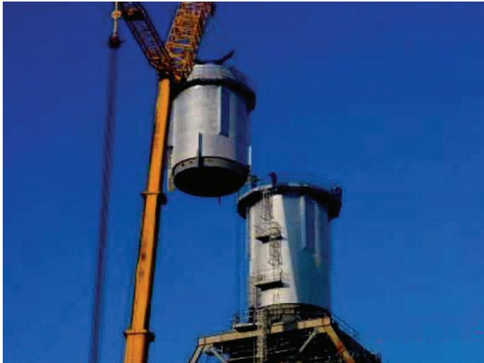
*Figure 7: The HRSG upper part stack lifting*
