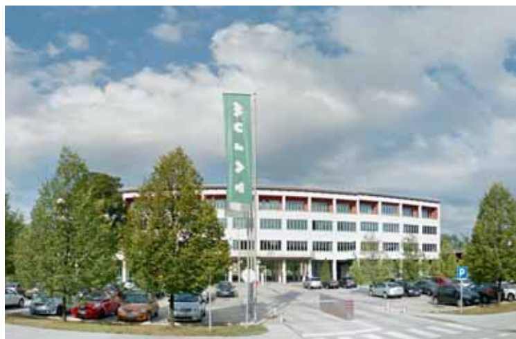
Google Street View, Talum 2013
