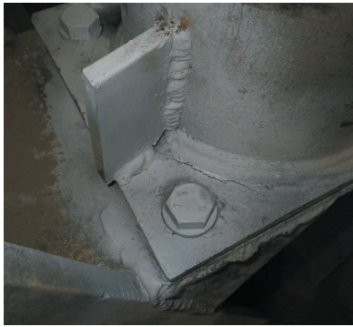
Fig. 3. Fatigue crack in the side bracing
