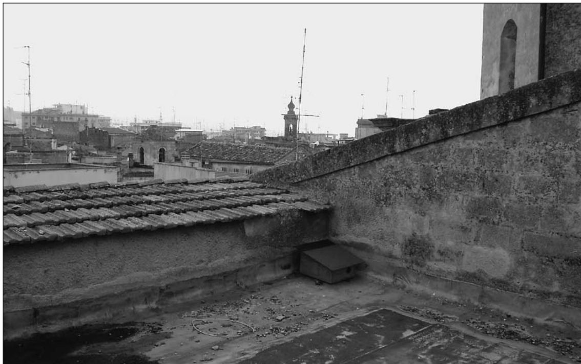
Figure 2: An example of a nest box for Lesser Kestrel Falco naumanni placed on the roof of a building
