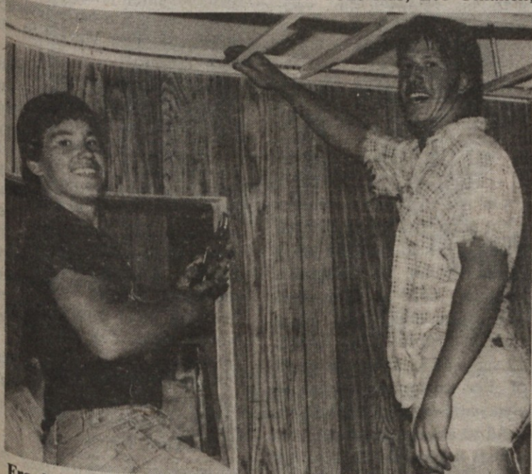
Frank Kogovsek Jr. (left) and Tony Rus lay supports for the lowered ceiling in the newly created front office.
