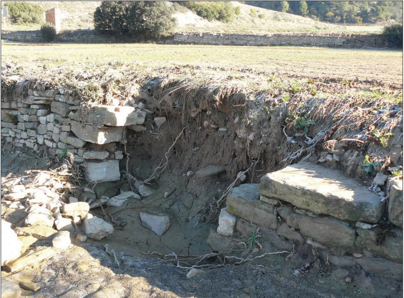
*Figure 7: Segment of stone wall on the floodplain of El Sió removed by a waterfall of overland flow produced by the storm of 2nd November 2015 (c. 75 mm in 3 h). Notice the volume excavated by the waterfall at the base of the missing segment of the wall.*
