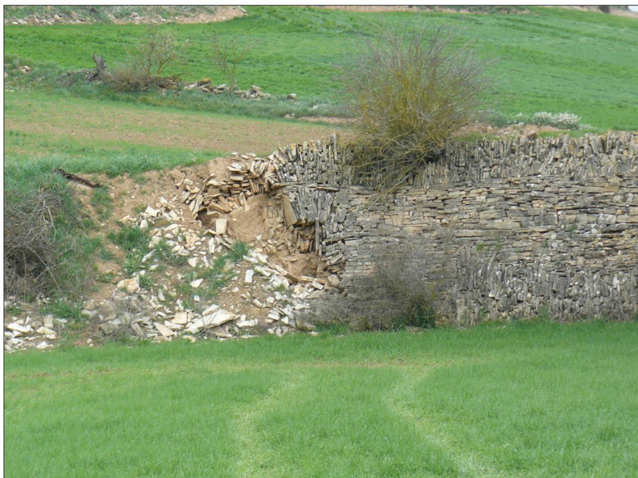
**Figure 2: Dry-stone wall with derelict segment (on the left) and standing segment (on the right) with three to four different patterns in the structure.**
