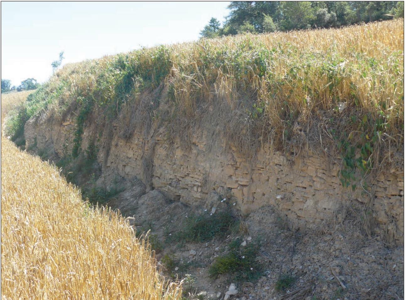
**Figure 5:** Stone wall not reaching up to the surface of the upper field. Notice soil sediments accumulated at the base.
