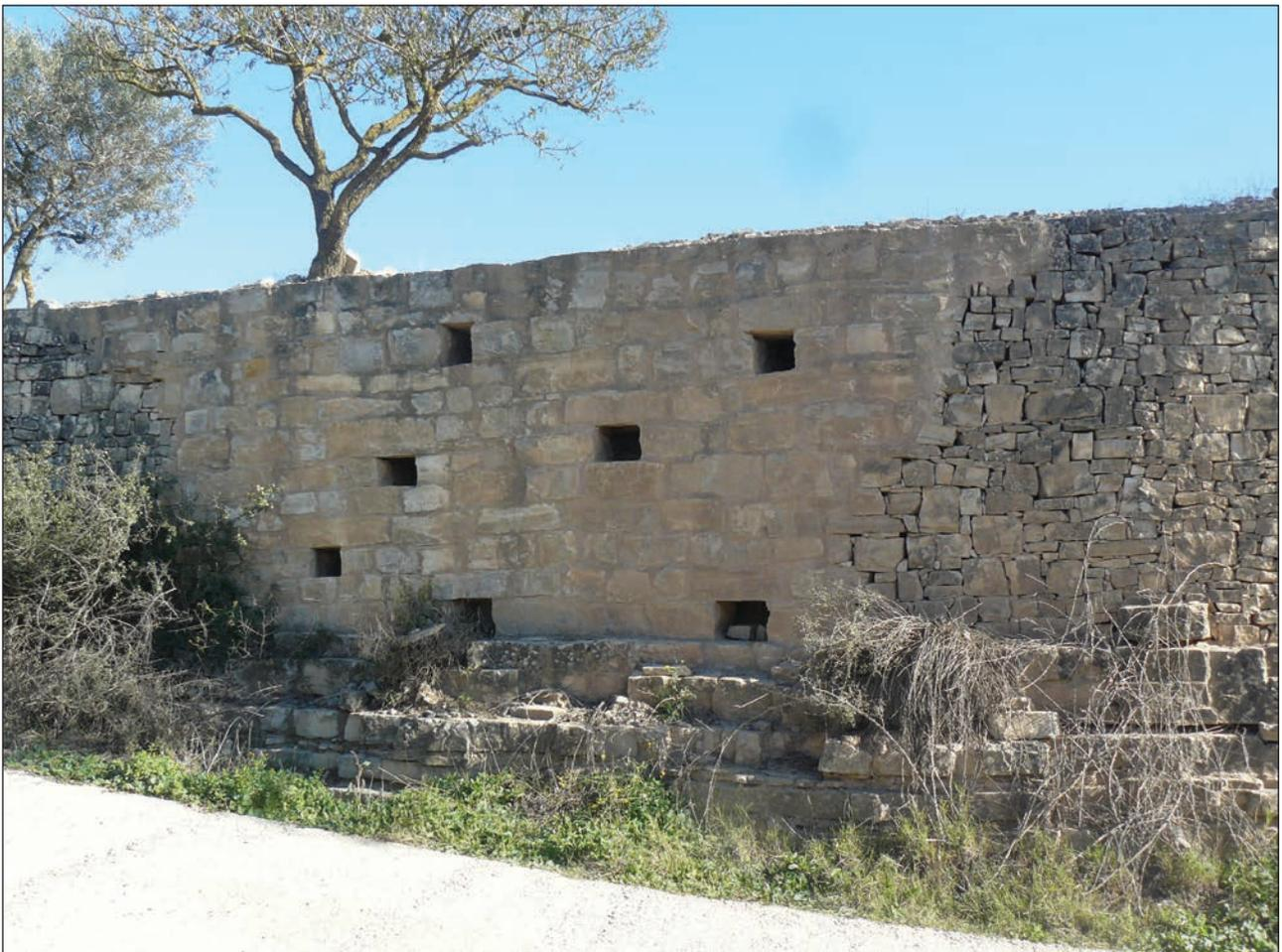
**Figure 3:** Stone wall built on a limestone outcrop with repaired segment on the left (notice drainage holes) and old segment on the right.
