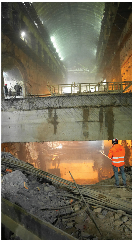
Figure 7: Powerhouse cavern under excavation of lower part.
