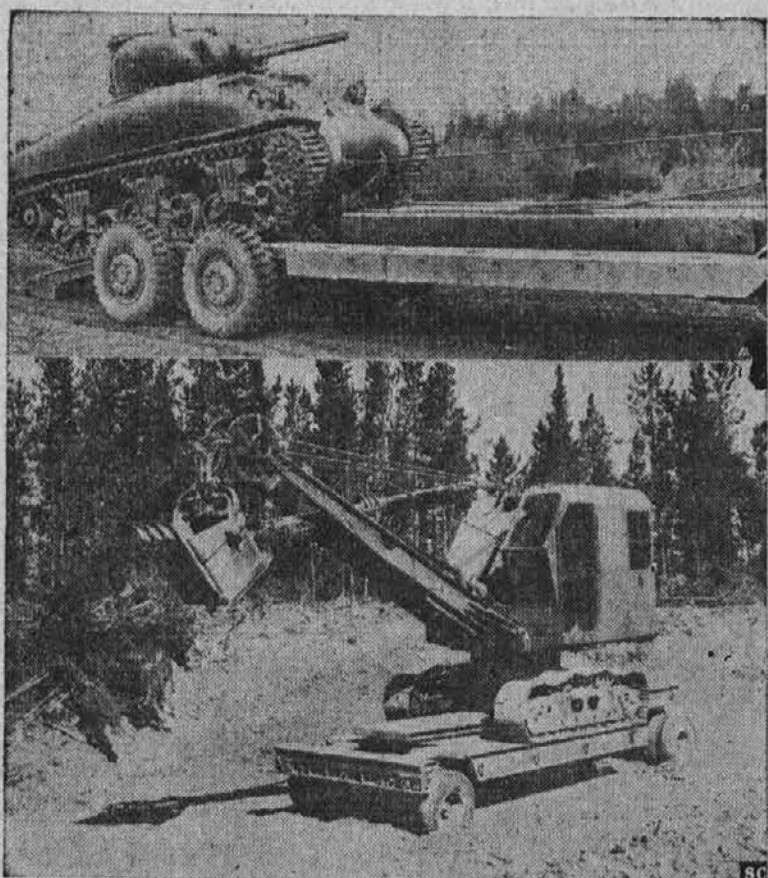
The big heavy-duty flat-bed Fruehauf Trailers which proved of such tremendous value in transporting heavy peace-time machinery are now proving their worth in war-time. The same type of trailer, with considerable equipment installed, are being used to haul fighting tanks to the front and to retrieve them when damaged by enemy fire or mechanical difficulty.
