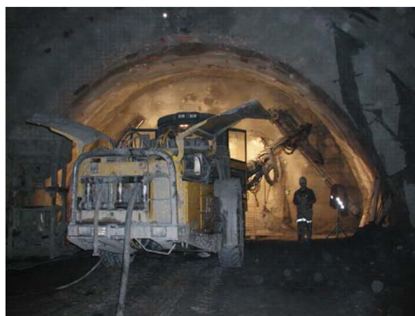
Figure 2. Installing micro piles into the side of the tunnel.
