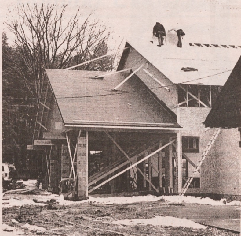
View of the new building from the playground.
