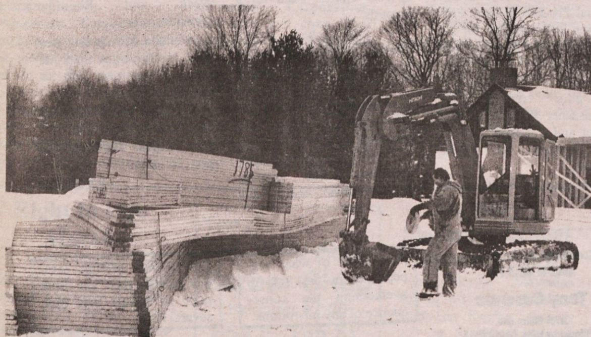
In charge of the project is quality builder Tom Znidarsic.
