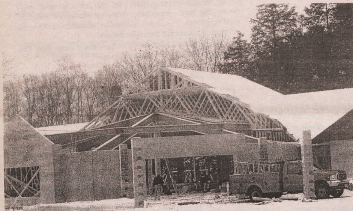
Despite the cold and snow, the roof of the new Slovenska Pristava building, goes up, even during winter, thanks to all the volunteer workers.
