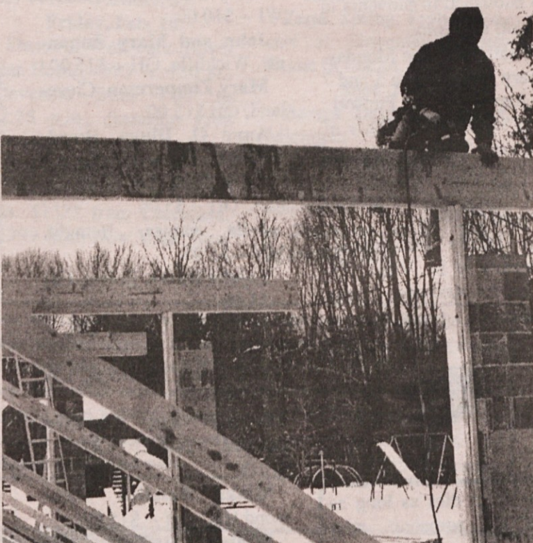
Freezing weather doesn't prevent Mike Rus from using the nail gun on the frame of the roof.
