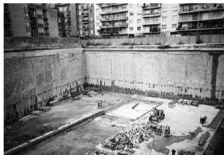
Gradnja, ki je potekala 22 metrov pod nivojem ceste in 11 metrov pod nivojem podtalnice. Vsakih pet metrov smo zgradili temeljne zidove, ki so v zemljo zasidrani z jeklenimi sidri. The construction 22m below ground, 11m under the water table. Every five metres, retaining walls were built with steel anchors into the earth.
