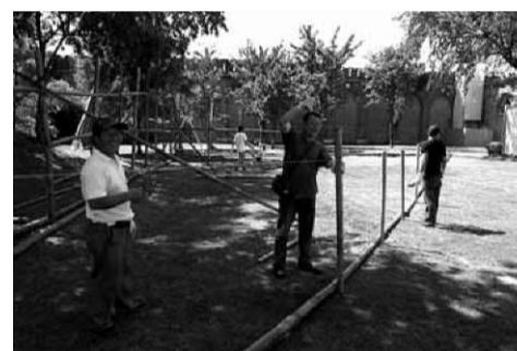
Gradnja v Benetkah. The construction process in Venice.
