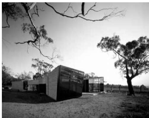
Vila Vinograd, Avstralija, dokončana 2004. Vineyard Residence, Australia, completed in 2004.
