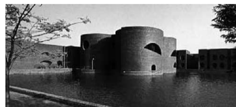
Pogled preko jezera na Narodno prestolnico Bangladeša; valjasta zgradba jedilnic z dvojnimi opečnimi stenami je v sredini, na desni pa so prenočišča. View across the lake to the Bangladesh National Capital; the cylindrical, double-shell brick dining halls are in the centre and the hostels are on the right.
