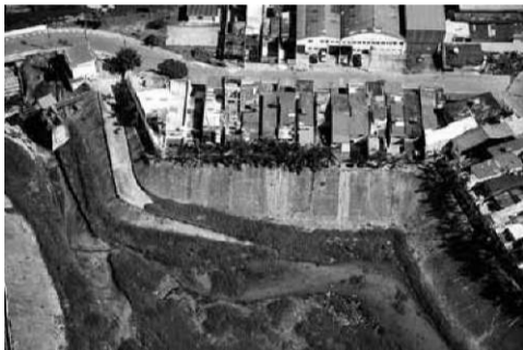
Rezervoar, postavljen tik ob hišah. Reservoir placed right next to people's houses.
