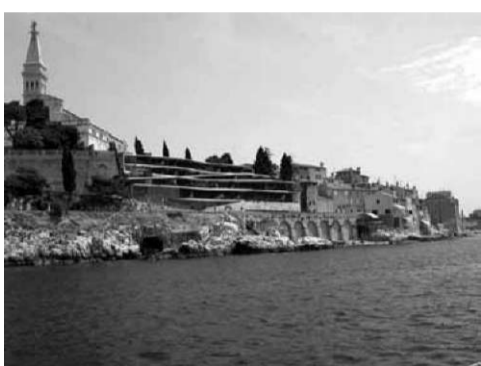
Hotel Rovinj, Rovinj, natečajni projekt, 2007, pogled z morske strani. Hotel Rovinj, Rovinj, competition project, 2007, view from the seaside.
