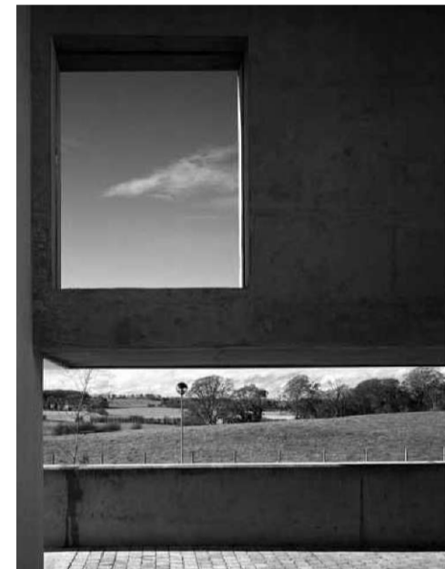
Vhod v šolo, spodnji pogled ven uokvirja pokrajino, zgornji pa nebo. Spreminjanje barve in podobe neba sta pod nadzorstvom arhitekture. The entrance threshold where the lower view is about framing the landscape and the upper view is framing the sky. The changing colour and the character of the sky are monitored architecturally.
