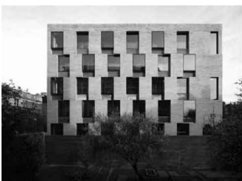
Zahodna fasada, 450 mm debel zaslon, ki daje občutek debeline kamna. The west elevation, the 450mm deep screen, which makes you feel the depth of the stone.
