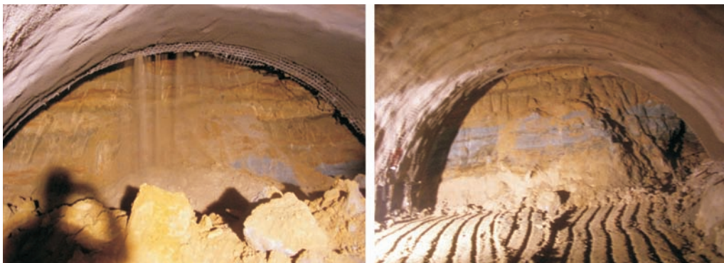
Figure 11. Flow of sand from the ceiling of the top heading (BT8) in the right tube at the ch. 21672 (a) and the top heading in the right tube at the ch. 21659 (b), which indicates consequences of shallow shear overbreak due to discontinuities (BT3) on the right side of the excavation face.
