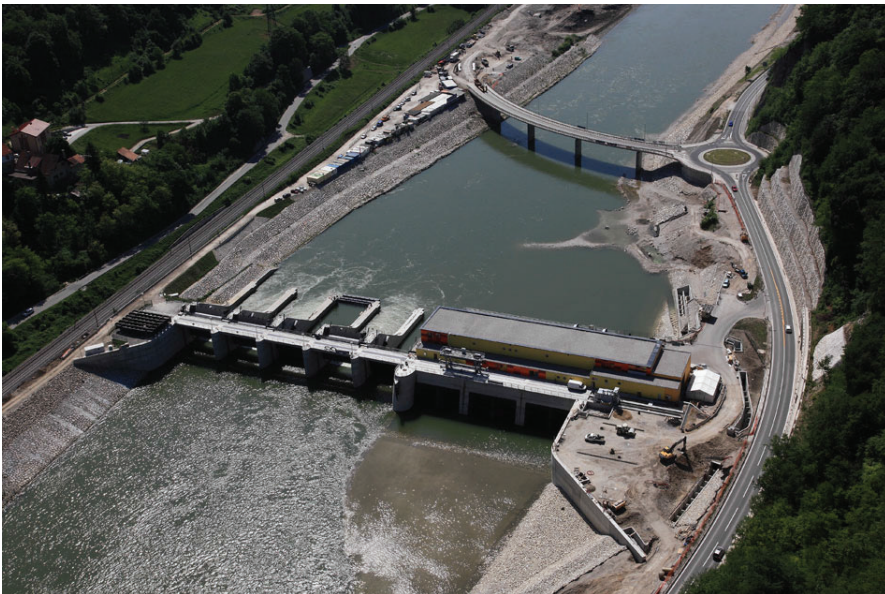
Figure 3: Krško HPP (photo Litostroj Power archive)
