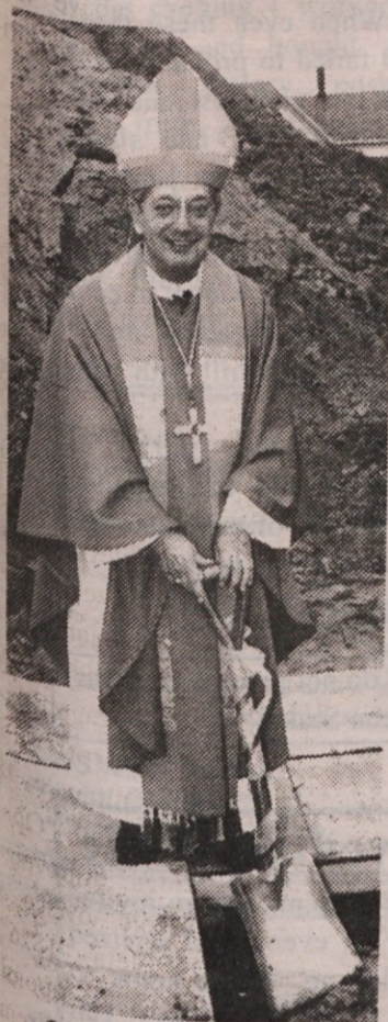
Cleveland Bishop Anthony M. Pilla gets ready to dig the first shovel of dirt for the St. Vitus Village.
