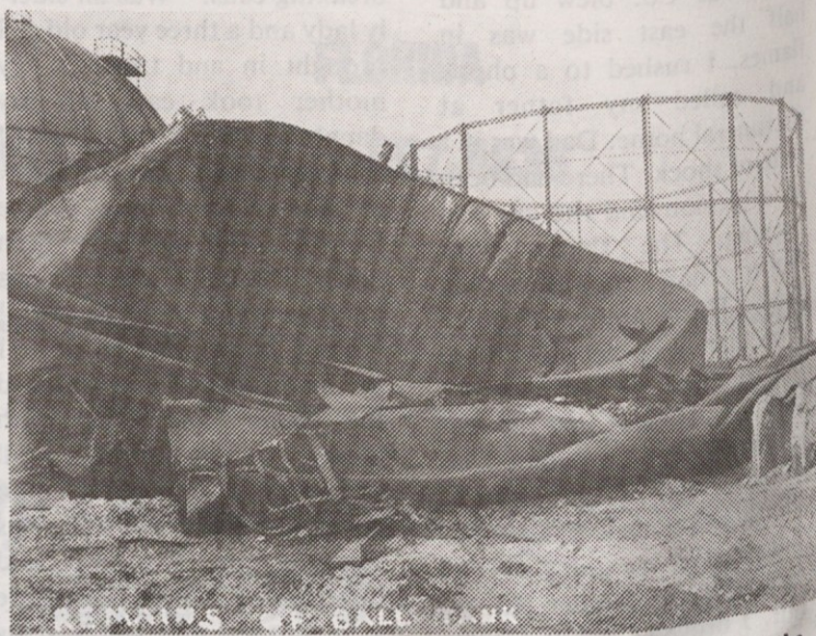
Shown is all that remains of the cylindrical tank (right), and the collapsed ball tank.
