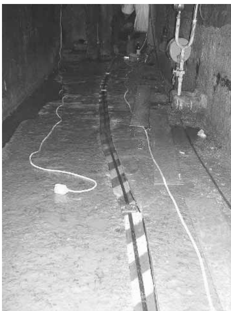
Fig. 18: SMARTape installation in the inspection gallery
