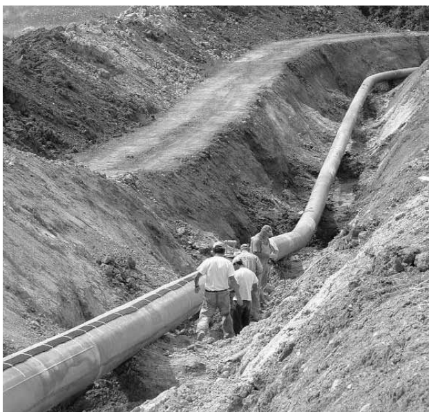
Fig. 19: SMARTape on the gas pipeline.
