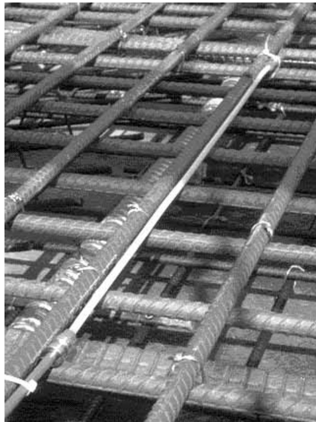
Fig. 3: SOFO Sensor installed on a rebar
