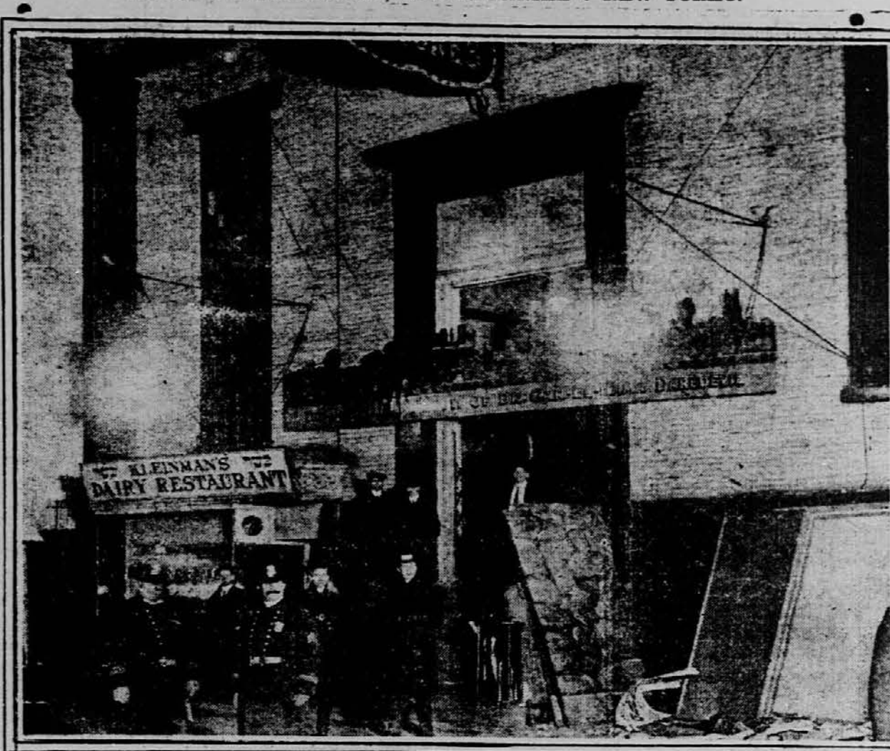
MOVING PICTURE THEATRE WHERE FIRE PANIC OCCURRED.
