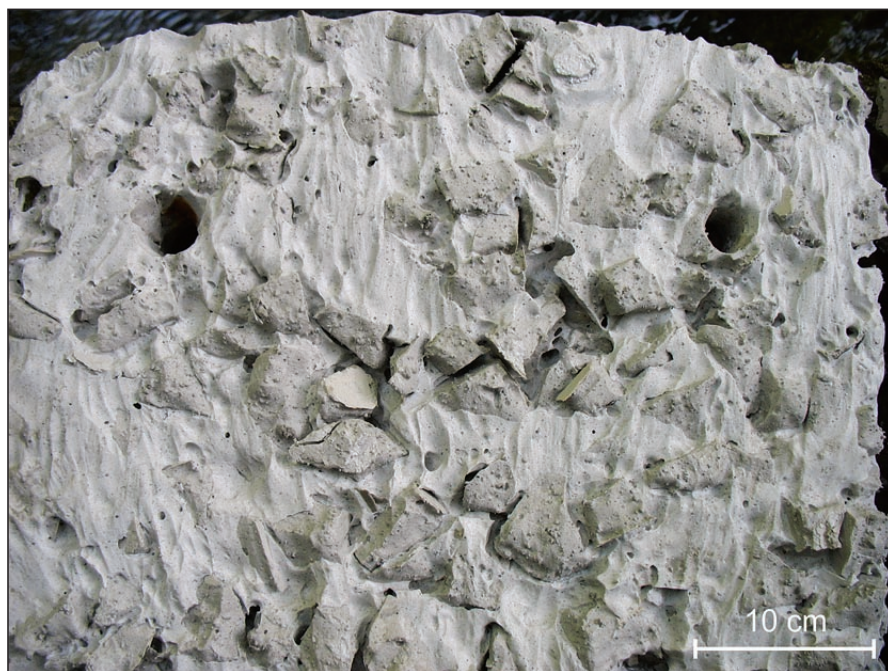
Fig. 17: Channels and pockets in plaster layers with harder fragments.
