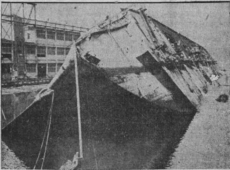
S. S. Lafayette (Normandie) was floated off mud recently and passed critical point in salvaging operations, righting to an angle of
