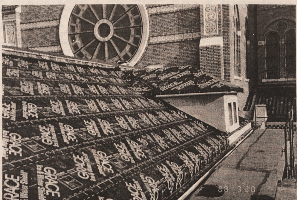
Ice and water guard protection is being installed over the entire rectory roof that will have new clay tiles.
