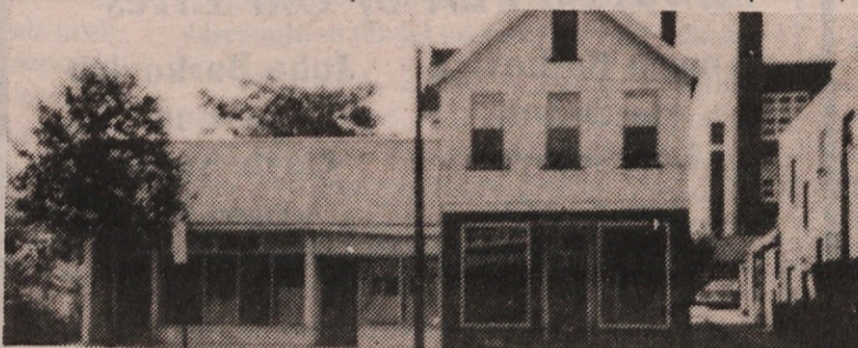
The Jablonski-Svete stores at 6120-22 St. Clair before being razed in 1981. (Photo by Vince Gostilna)
