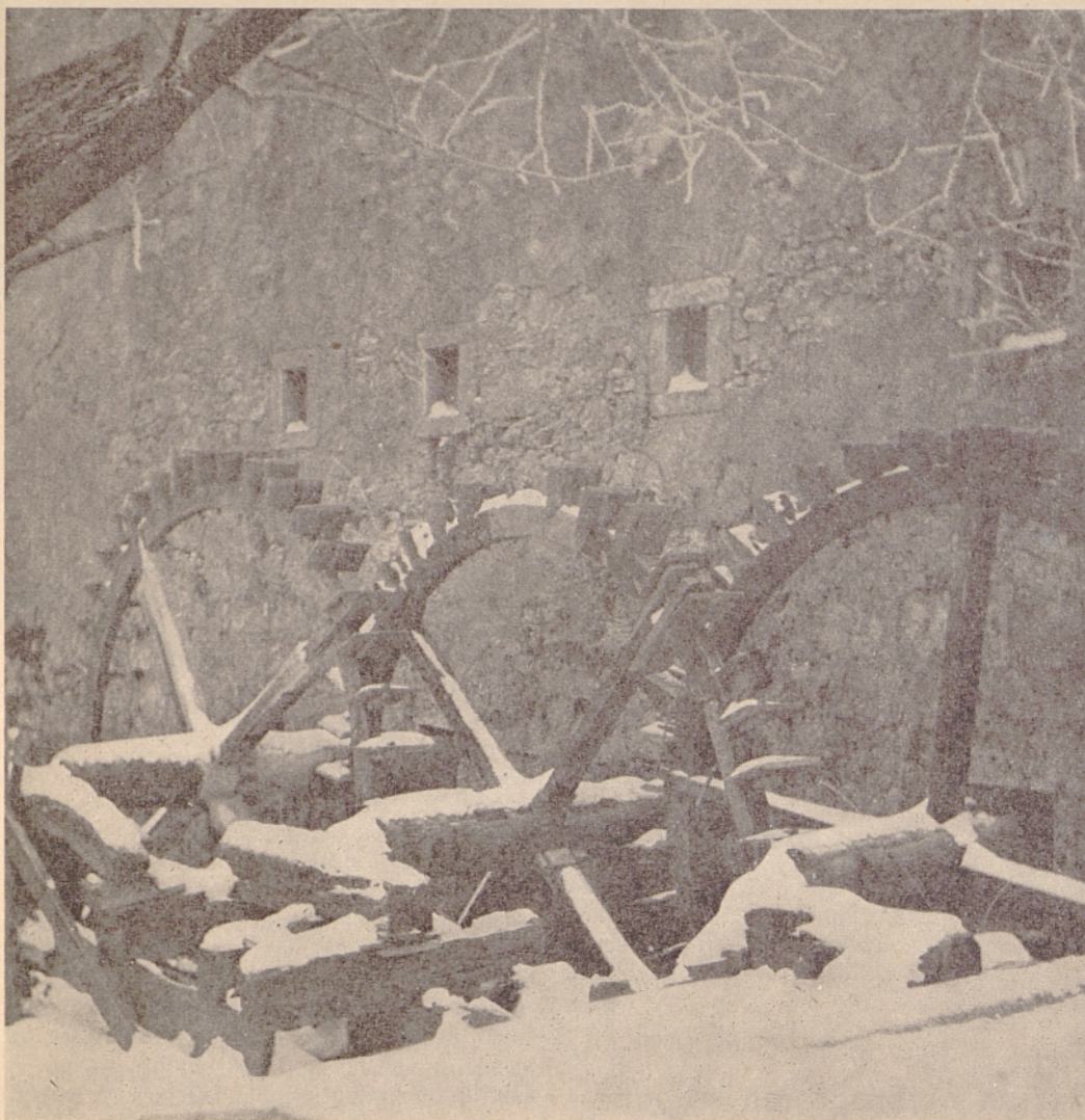
And old mill covered with snow
